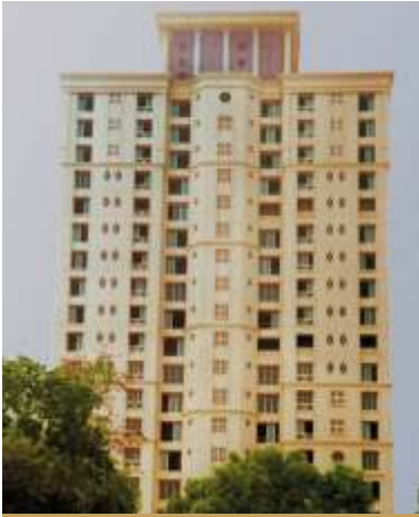
Carlton Building, Thane
