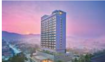
HVAC Installation for Taj Hotels & Resorts
