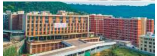
Chiller installation for Symbiosis Hospital Pune (900 beds)
