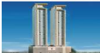
HVAC for AJMERA Aeon & Treon towers
