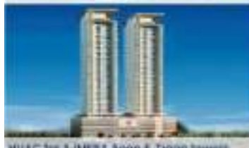
HVAC for AJMERA Aeon & Tiran towers
