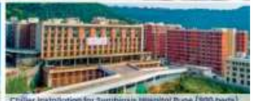
Chiller installation for Syntiposis Hospital Pune (300 beds)
