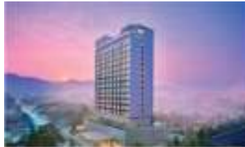
HVAC installation for Taj Hotels & Resorts
